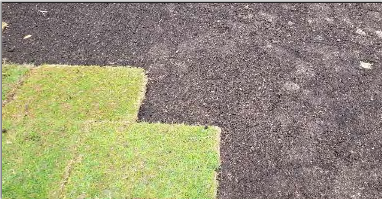
The soil at this site has been properly cultivated and the installer is laying the sod in a brick pattern.
